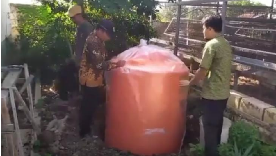
Figure 4. Biogas Initial Installation
